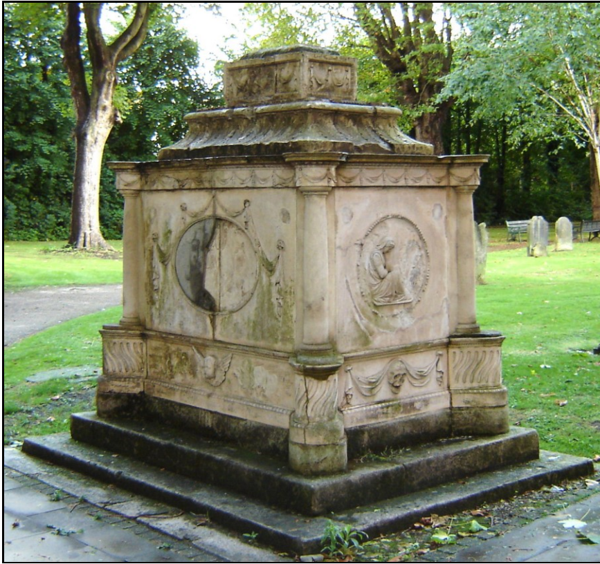
The tomb of Harriet Thomson made of Coade artificial stone in the Putney Old Burial Ground on the Upper Richmond Road. (Philip Evison)
